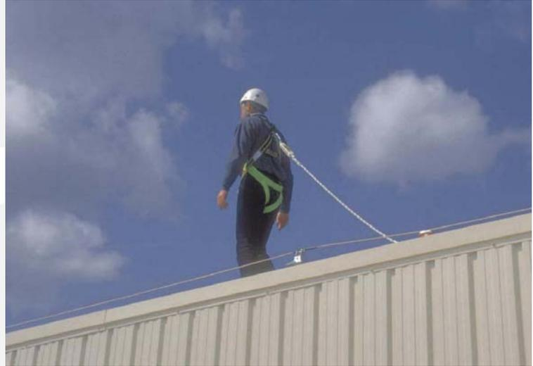
In addition, Xenon allows users to work at 180° of the lifeline without having to disconnect, or allows them to simultaneously work on both sides of a ridgeline, which improves the productivity of your teams.
